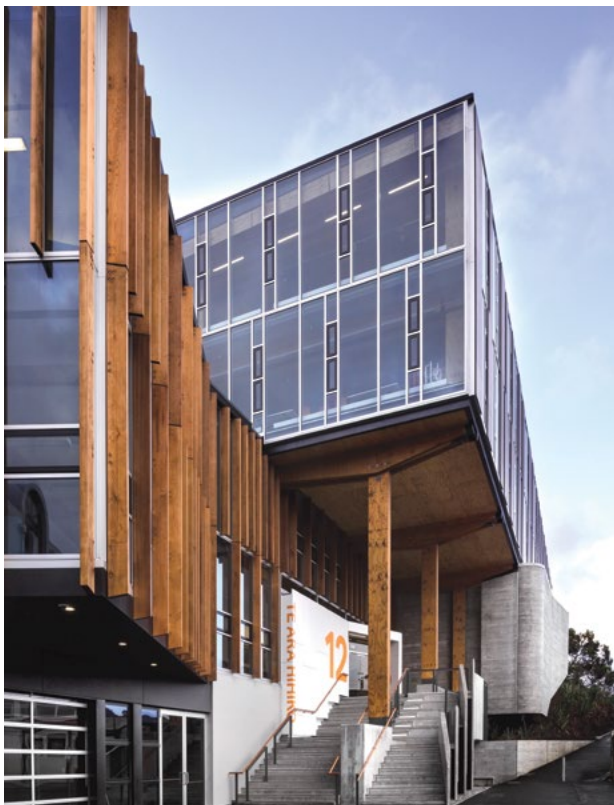
College of Creative Arts (CoCA), Wellington (maintained two coats of Drydens wood oil for exterior exposure),
